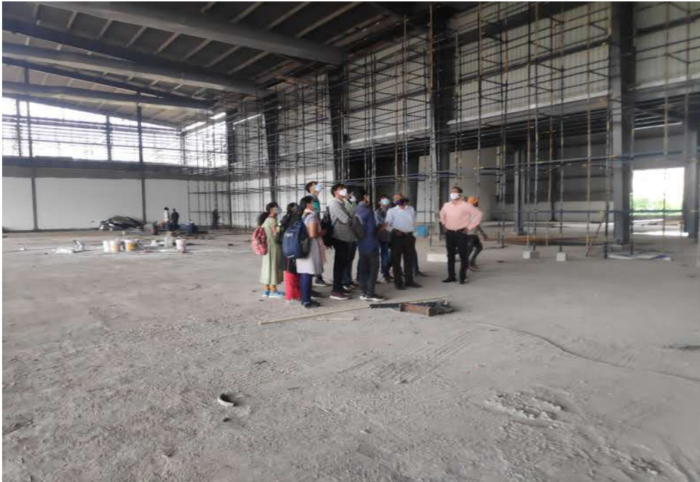
Students at construction of function hall using PEB structure at Bachupally
