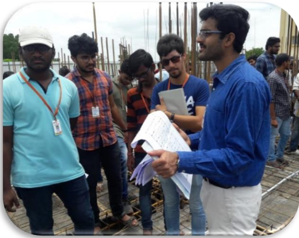
III B.Tech Students visit to VJ Hostel Building
