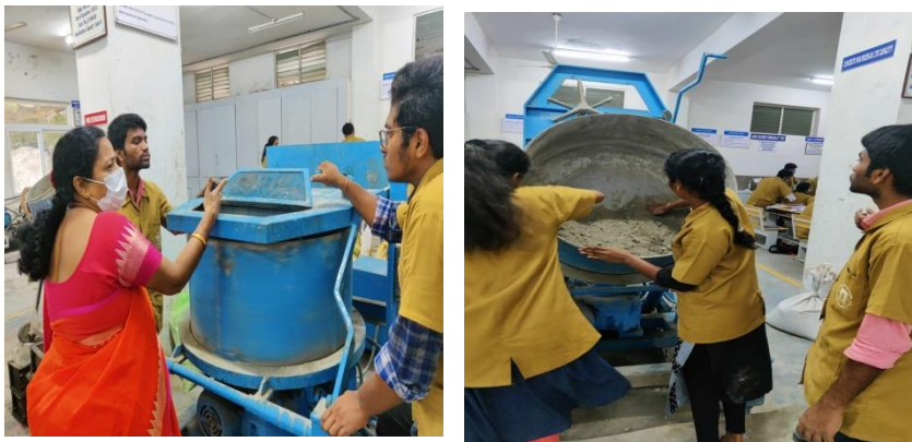
Fig: 1 Concreting of Self Curing concrete
