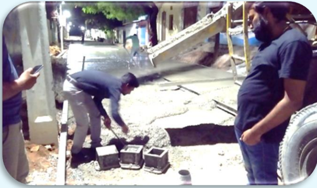
D. Anil Kumar collecting Concrete samples
