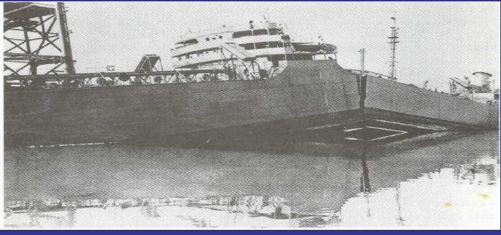
• Failure of Liberty Ships during services in World War II. Seven of the Liberty ships built during the world war II have failed completely breaking into two as a result of brittle fractures. Over 1000 of approximately 5000 merchant ships built during World War II had developed cracks of considerable size and became unserviceable.
