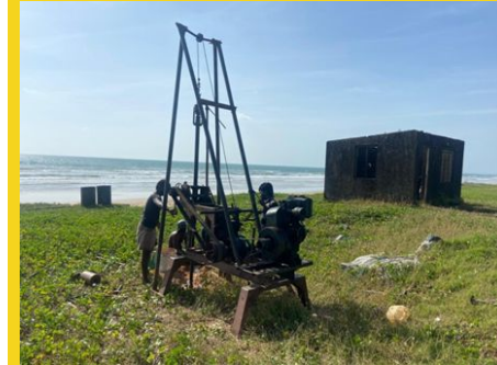
Geotechnical investigations at Koderi West and East (Byndoor)- Mangalore
