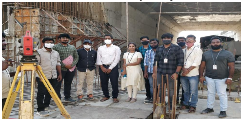
I M.Tech. (Structural Engineering) students at the construction of Railway under Bridge along with the faculty of CED, VNRVJIE on 24.12.2020
