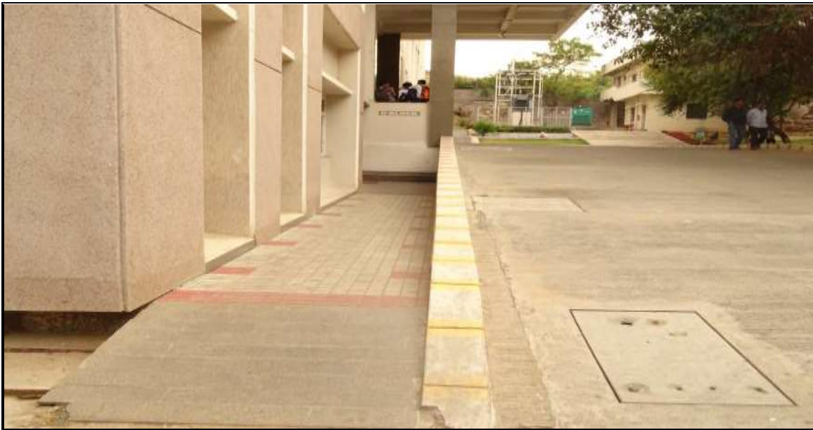
Ramp way 2 in the entrance of Yogiah Naidu Bhavan
