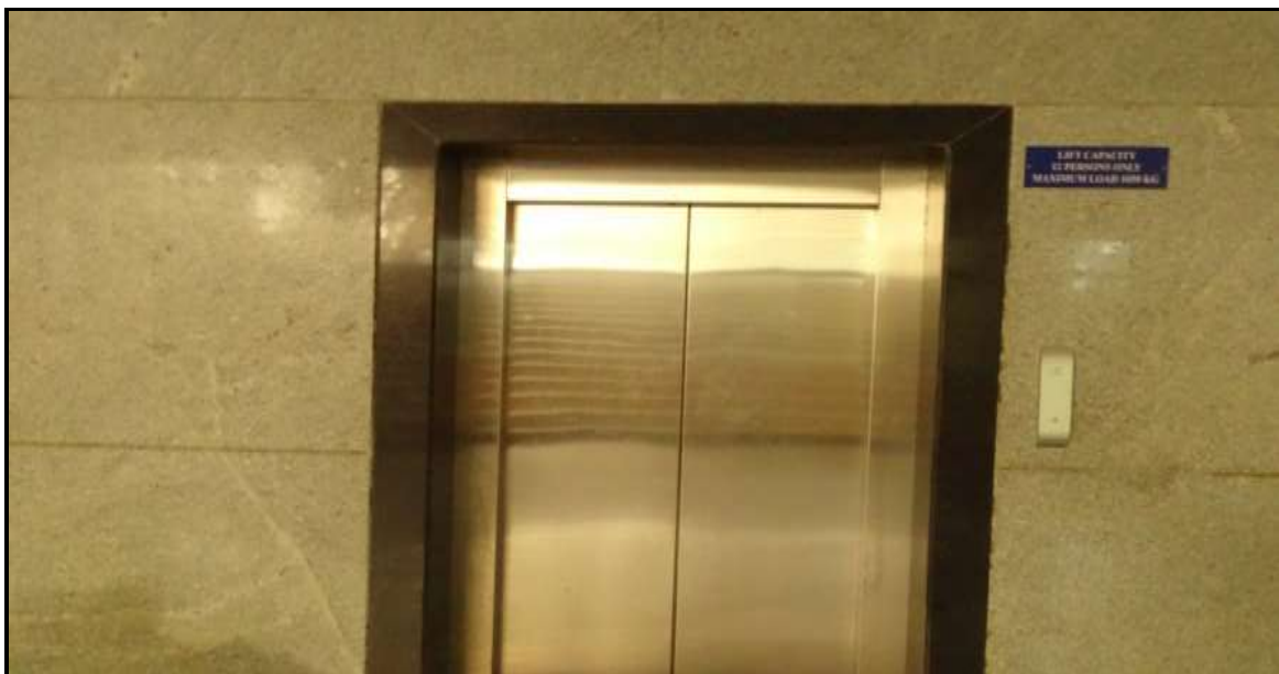
Lift 4 in Yogiah Naidu Bhavan of 12 Persons capacity
