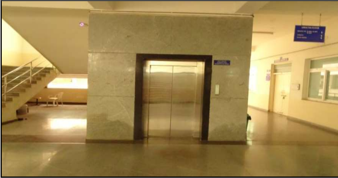
Lift 5 in Yogiah Naidu Bhavan of 12 Persons capacity
